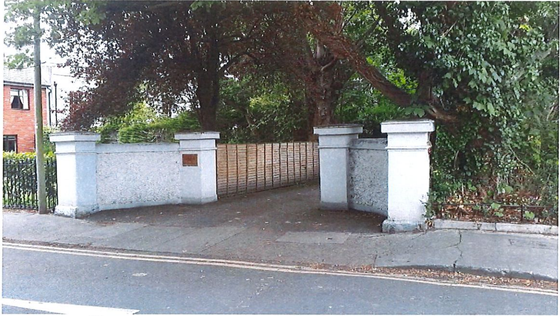
Shared entrance gates for 28, 27a & 28 onto Oakley Road
