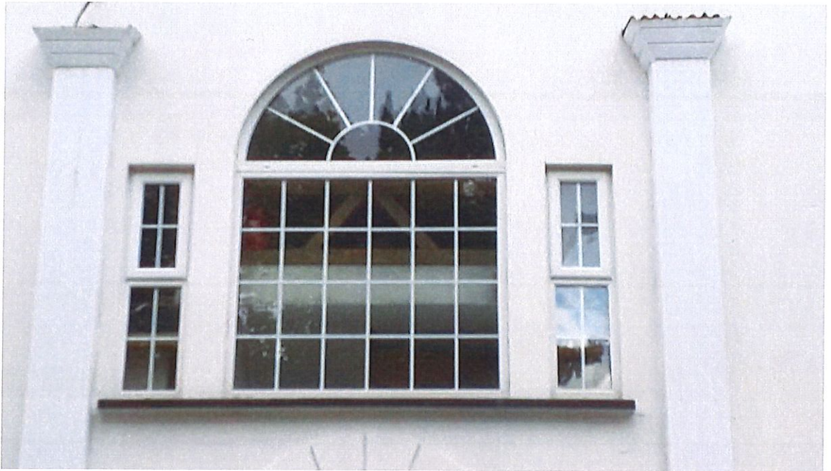
First floor uPVC 'Wyatt style' window
