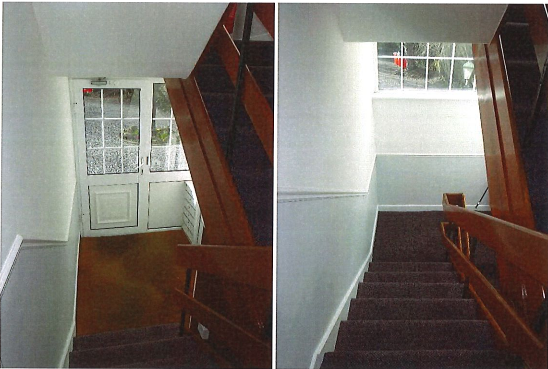
Main modern concrete staircase at ground floor level
